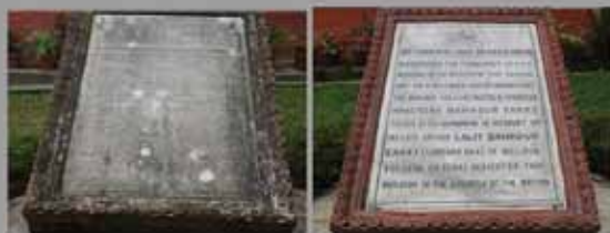
Foundation Stone before and after renovation by students .
